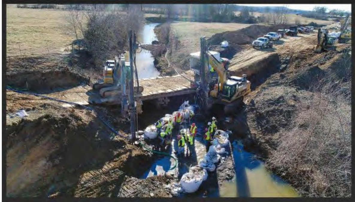
Arkansas 2017 – Pipeline Blasting - Dykon Blasting
