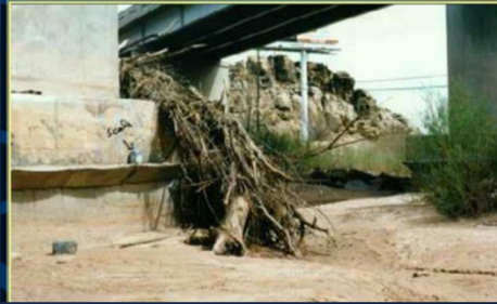
Field Evidence Of Long-Term Scour
